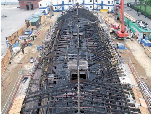
An aerial image of the main deck showing the extent of the fire. It remains to be seen how much damage the ironwork has sustained
