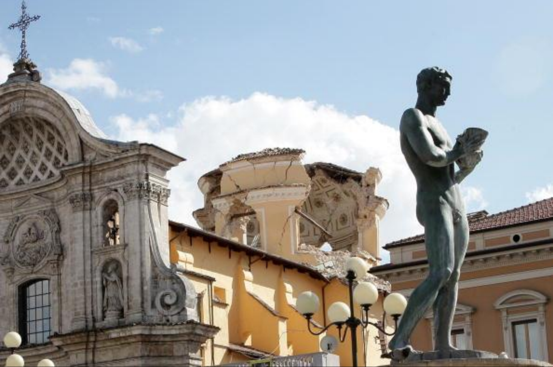
L'Aquila earthquake : 6 April 2009
