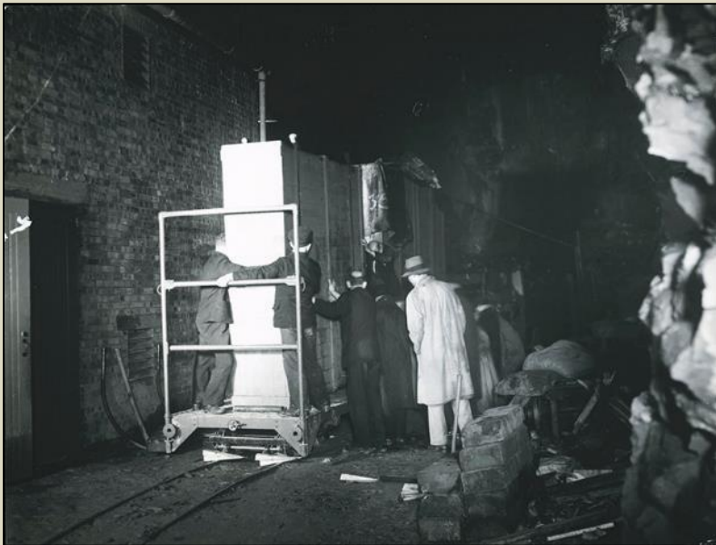
Unloading cases at the quarry entrance, February 1943. ©The National Gallery London
