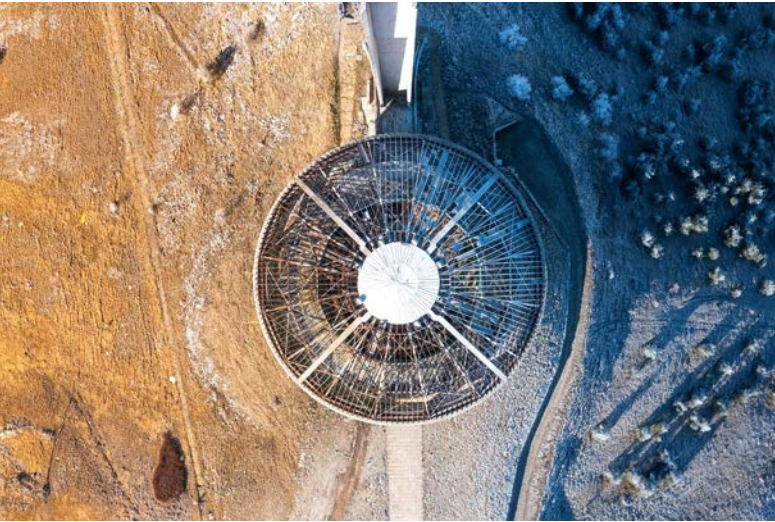
The cleared roof with the completed protective shelter over the dome mosaic. Drone photo by Alexander Makedonski.
