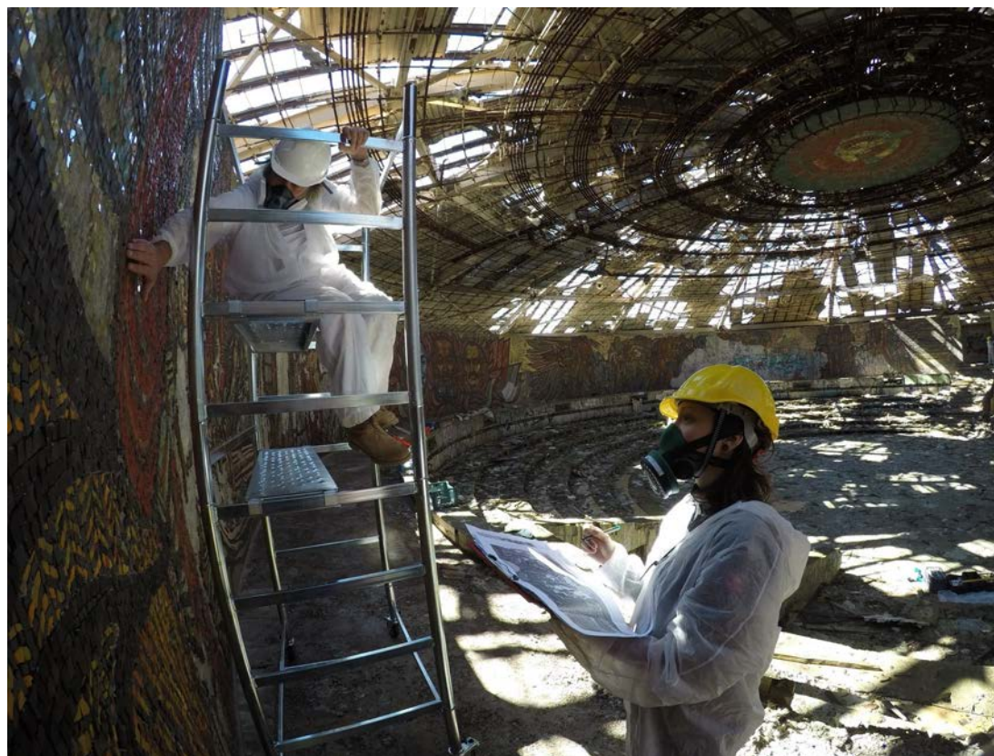
Deterioration mapping of the wall mosaics. Photo by Dora Ivanova.
