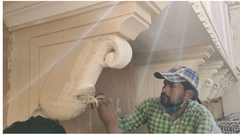
Left: Innovative storage and ventilation system adopted at the City Palace Museum, Udaipur. Right: Traditional lime plastering technique—Araish—still practiced at the City Palace Museum, Udaipur. All images courtesy of The City Palace Museum, Udaipur ©MMCF
