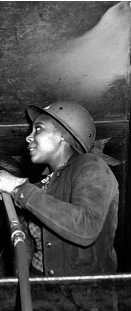
Center left: Kaiser shipyards, Richmond, California. Miss Eastine Cowner, a former waitress, is helping in her job as a scaler to construct the Liberty ship SS George Washington Carver. Photograph by Joseph, E. F. (Emmanuel Francis), 1943. Library of Congress Prints and Photographs Division Washington, D.C. 20540 USA http://hdl.loc.gov/loc.pnp/pp.print . Image reproduction number: LC-USW3-028673-C (b&w film neg.) Original location here .
