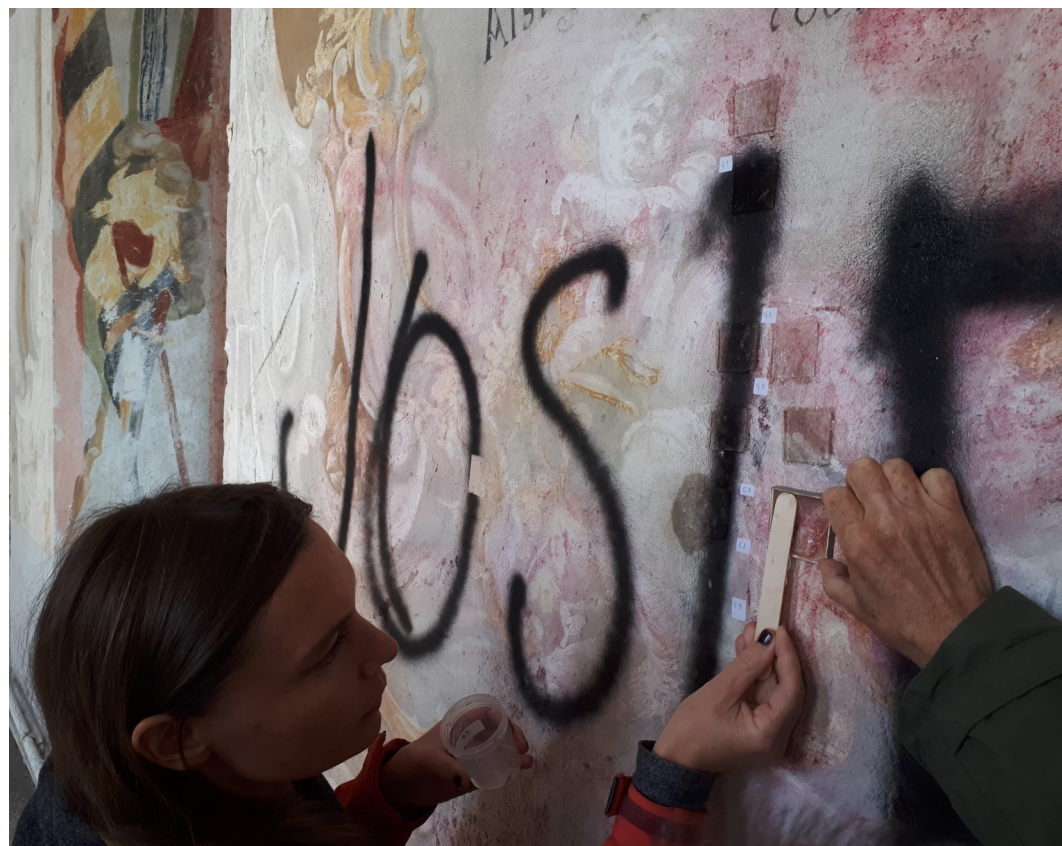
Martina Lesar Kikelj and Prof. Coladonato performing cleaning trials on graffiti paint with gels in Brezovica castle. Image taken by Neva Pološki.
